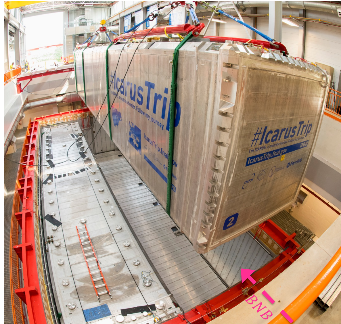
One of the ICARUS TPCs being lowered into the cryostat at FNAL, c. 2018
