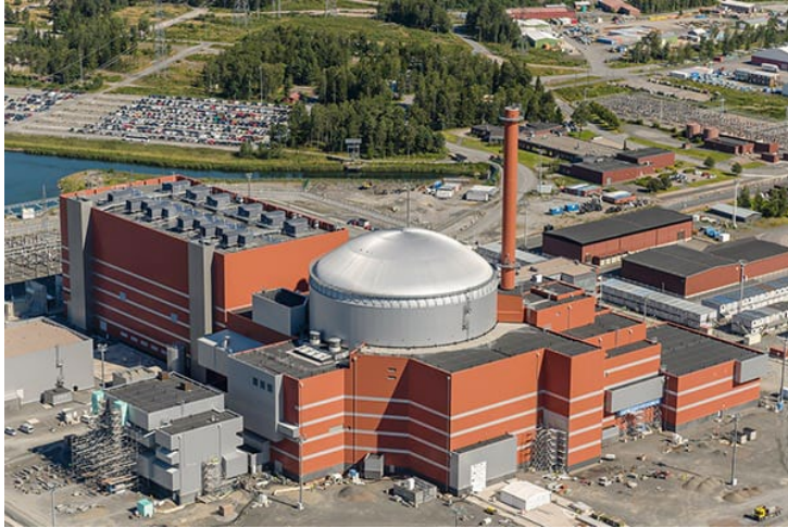
EPR (Framatome) in Olkiluoto (FI), 1600 MW
