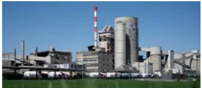
CO 2 -neutral concrete production
