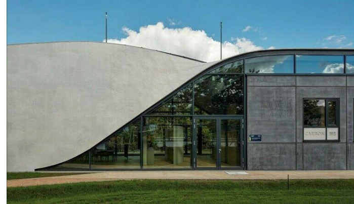
Example: Cube in Dresden - the world's first building made of carbon concrete (from: www.bba-online.de/news/cube-neues-bauen-mit-carbonbeton/#slider-intro-1 )
