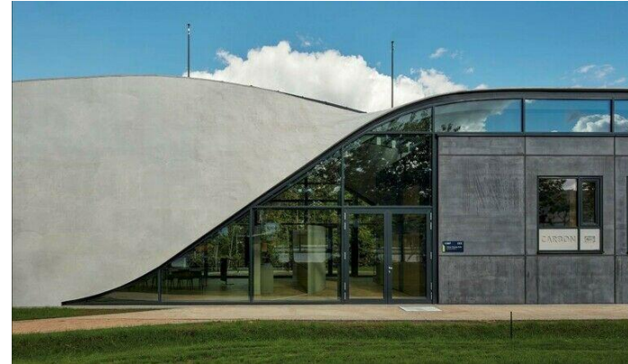
Example: Cube in Dresden - the world's first building made of carbon concrete (from: www.bba-online.de/news/cube-neues-bauen-mit-carbonbeton/#slider- )
